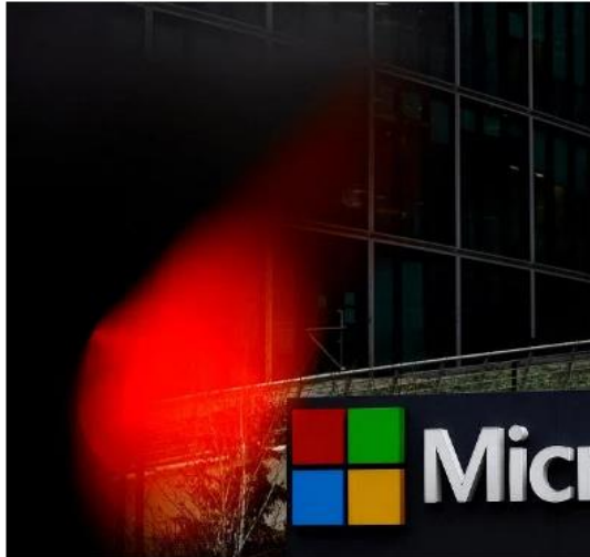
Microsoft said power was restored to the affected infrastructure in its data centre after temperatures returned to normal operating limits. PHOTO: REUTERS
